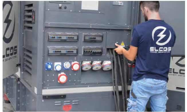
Power Terminal Box for cables with eye, it avoids damage to the contacts of the switch
