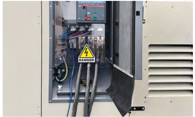
Power Terminal Box for cables with eye, it avoids damage to the contacts of the switch
