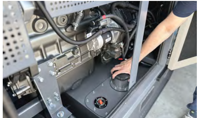
Tank filler with wide tank refilling point
