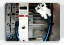
An **automatic circuit breaker** is mounted on the regulation circuit to protect against overload and short circuit on the voltage regulator.
